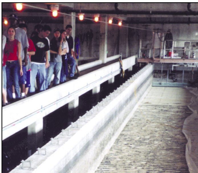
UCLA environmental science students get a rare view of an uncovered sand filter at the Tillman plant.
