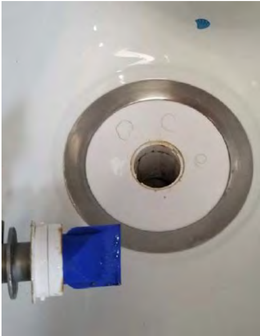
Figure 2 - Silicon Check Valve (6 Months)
