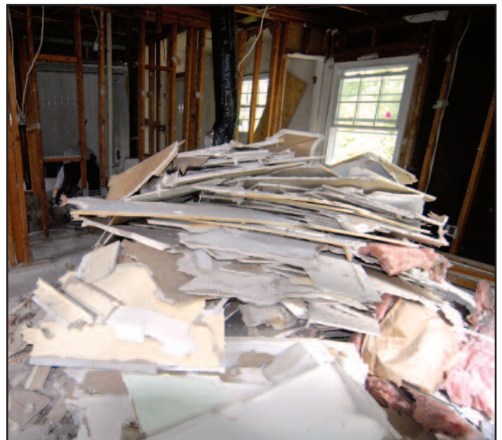
Rather than loading directly into dump trucks, workers carefully pile wood, wallboard and other debris so it can be sorted and evaluated for reuse.
