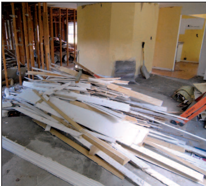
Rather than loading directly into dump trucks, workers carefully pile wood, wallboard and other debris so it can be sorted and evaluated for reuse.
