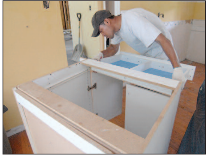
Modular cabinets can be taken apart step-by-step and reassembled elsewhere rather than going to a landfill.
